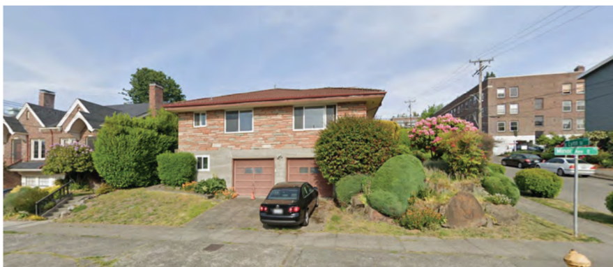
CURRENT 4-PLEX; VIEW FROM MINOR AVE E
