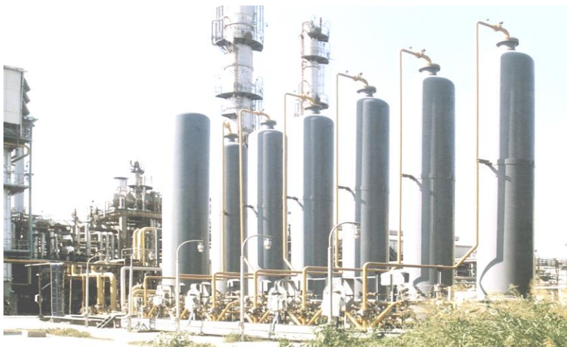
Figure 9.9 – Industrial sorption facilities
